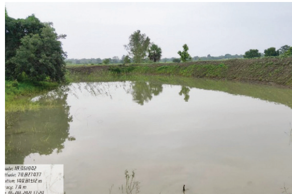
Water filled in OFR of Sri Kaveri Rajam
