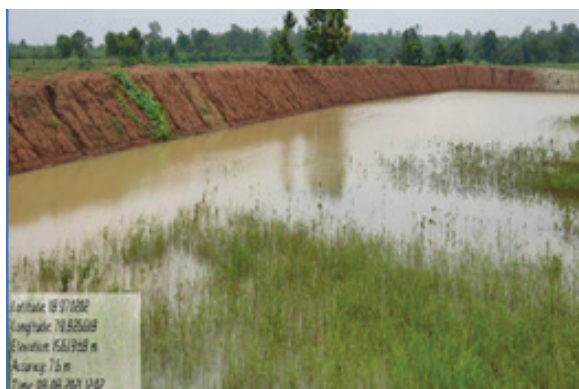
Water filled in OFR of Sri N Ammakka
