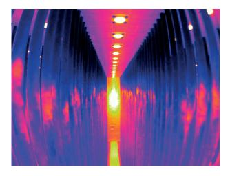
Figure 1. Thermal imaging of a top-fired SMR.
